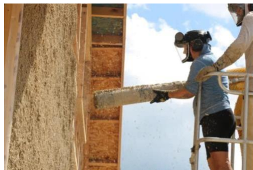
Figure 8 Hempcrete Formwork Installatio
