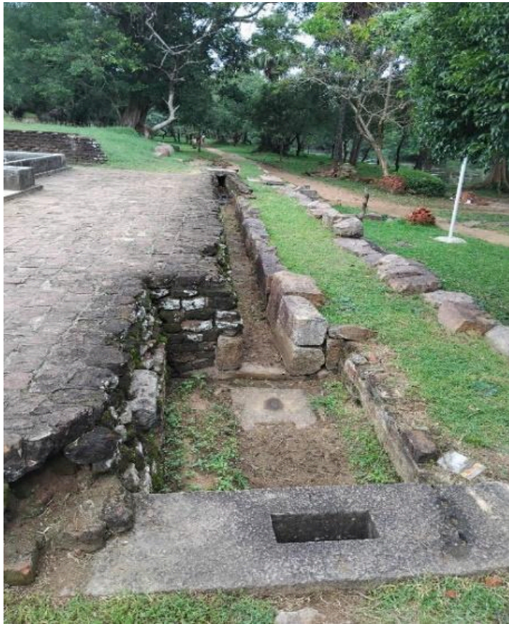
Figure 6. Water canal with a sluice gate made of stone
