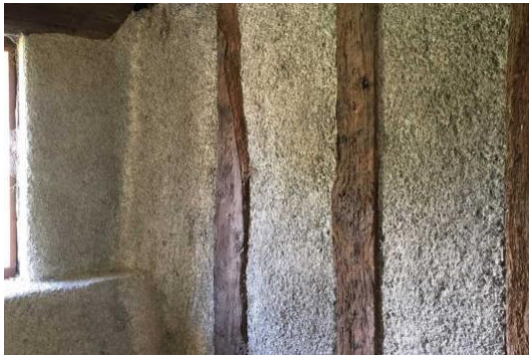
Figure 6 Hempcrete Wall- Infill
